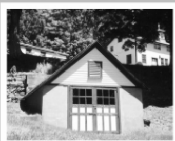
Valley Falls Farm - former ice house
