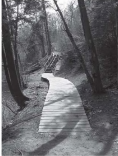
New boardwalk on Hemlock Hill Trail
