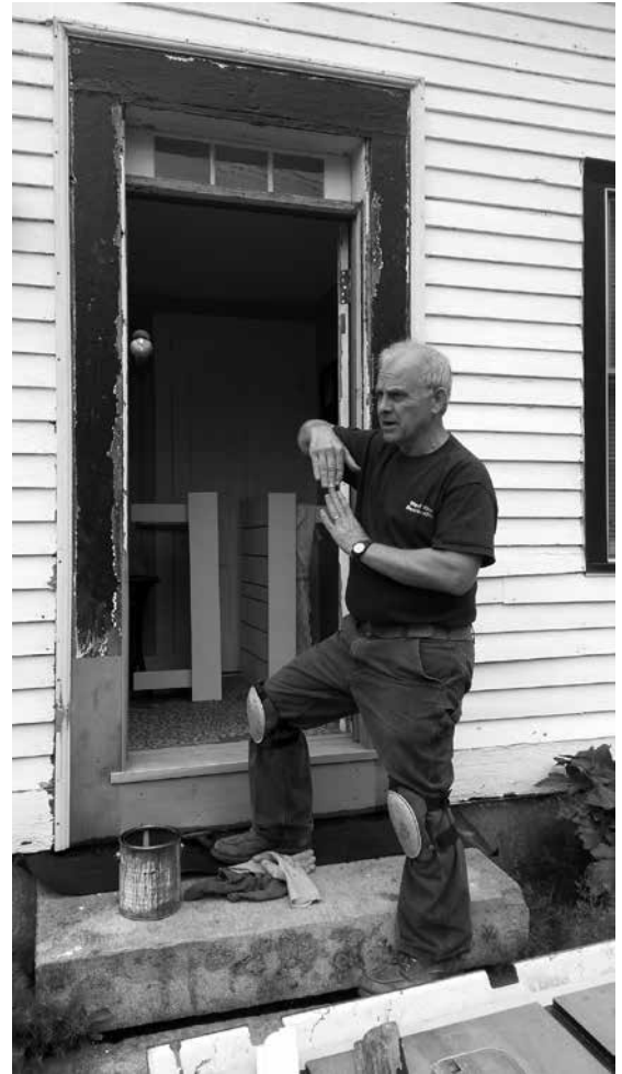
Restoration carpenter Tom Linskey restores the Valley Falls farmhouse door.
