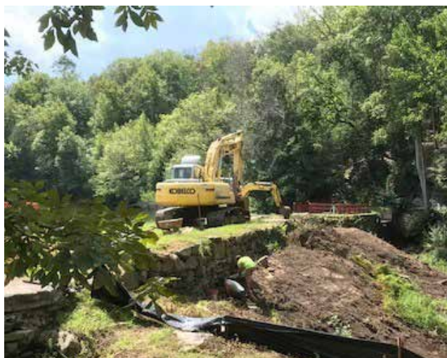
Dam reconstruction - photo by Karin James
