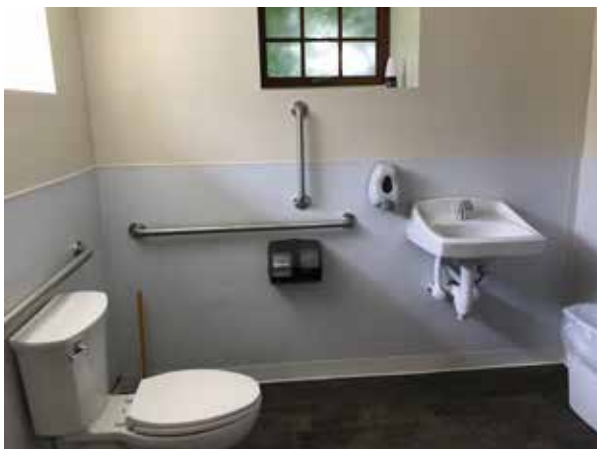
New Bathroom in the Red Barn! - photo by Karin James
