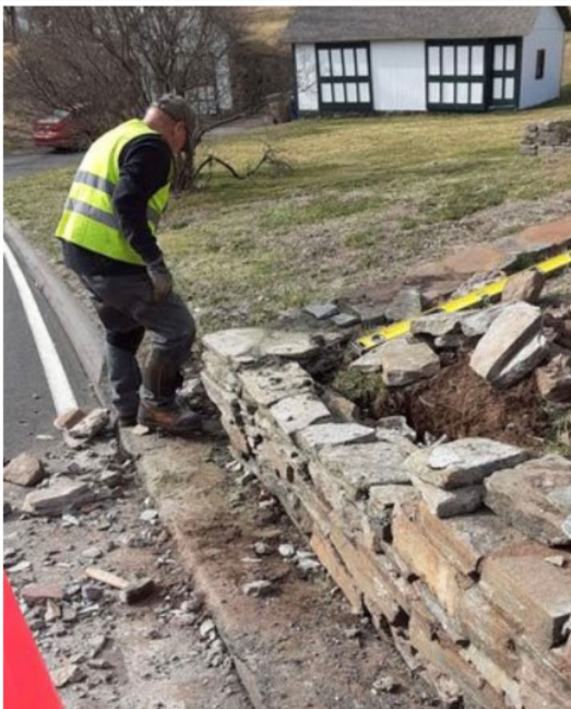
Ron Levesque fixes the damaged stone wall
