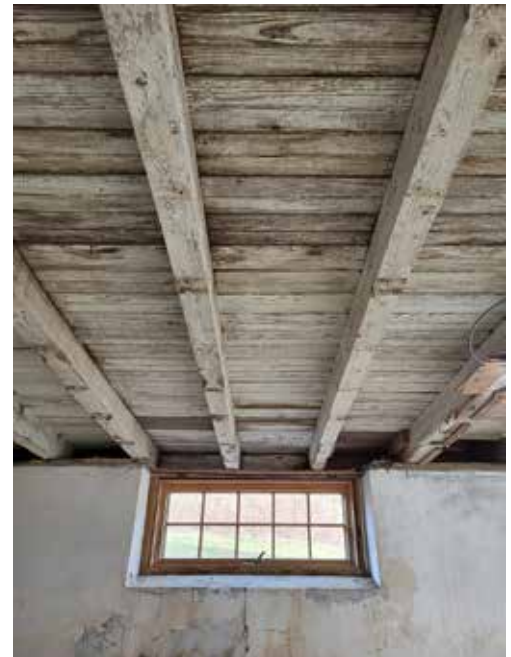
Exposed Beams. Photo by Ann Letendre.
